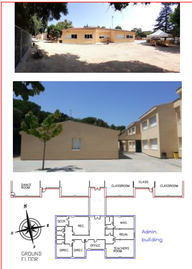
Fig. 2 The administrative building where the tests were carried out
